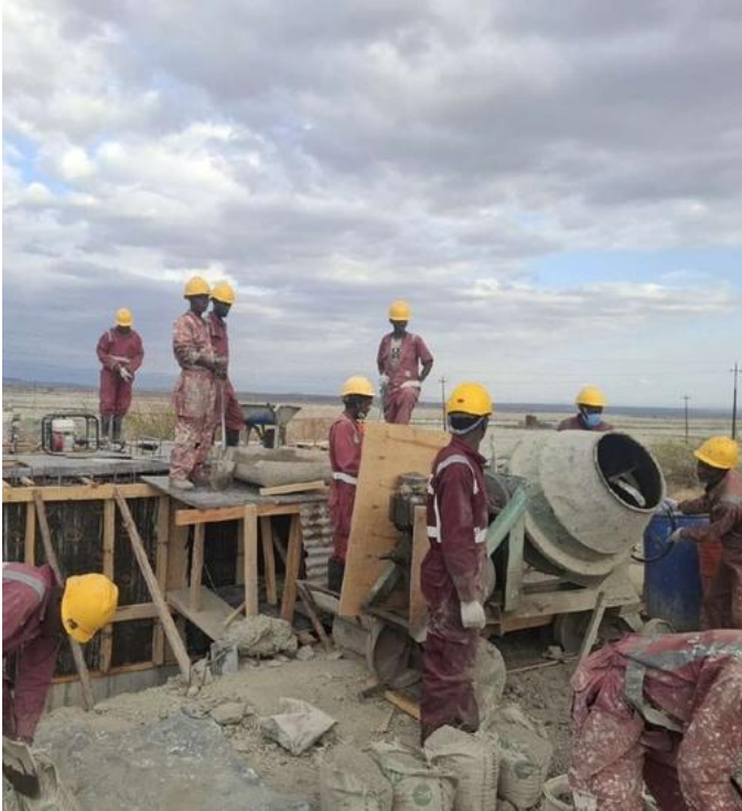
Dredge pump base / concrete placement
