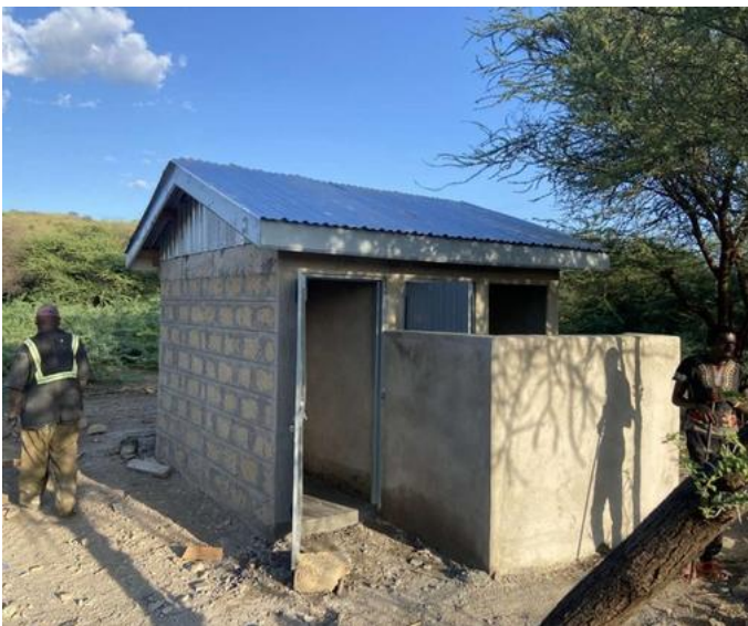
Lekishomi / community washrooms
