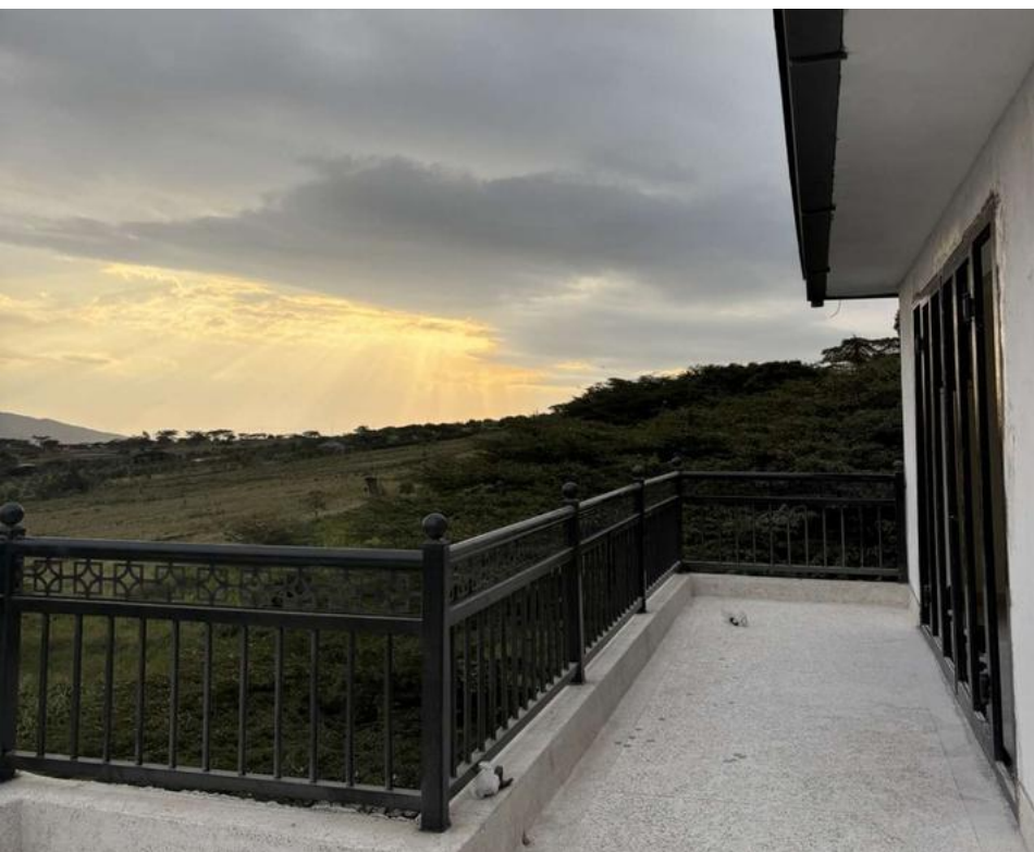
Kiserian / construction, bathroom finishes and terrace
