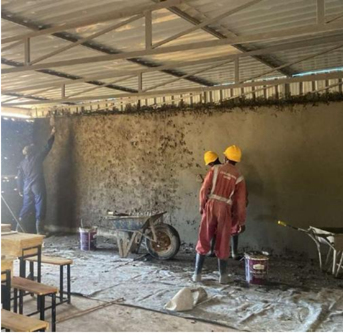
School refurbishment / work in progress
