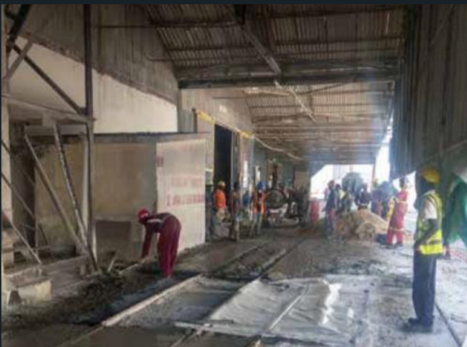
Railway works / industrial floor and track
