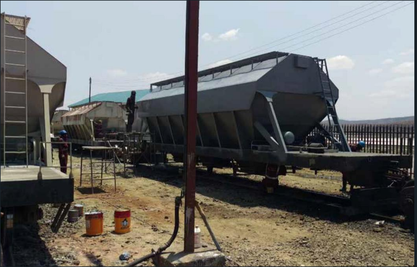
Hopper wagons / repair and painting
