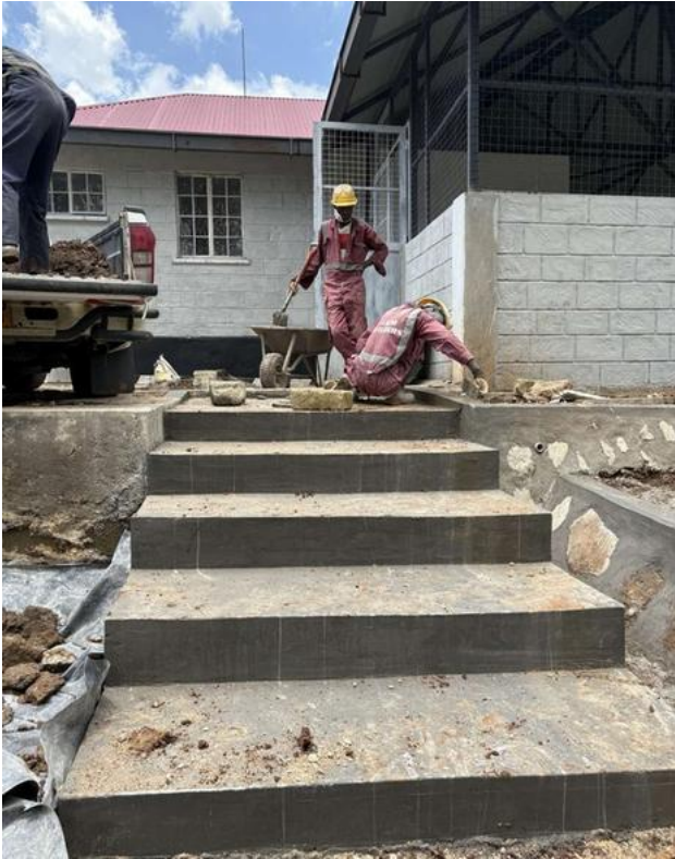
Central Hospital / access and building works
