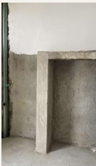
Interior repairs and room finishes
