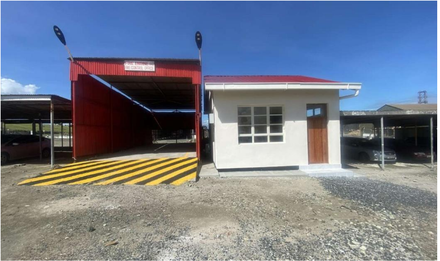
Fire station / office and truck shed
