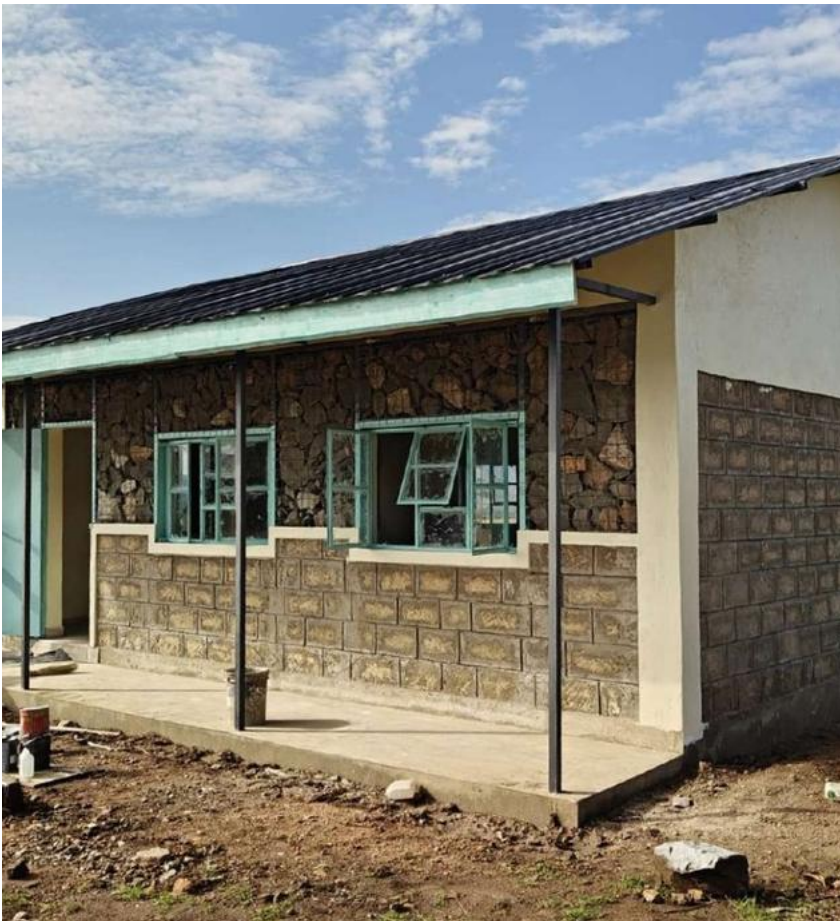
School renewal / external works
