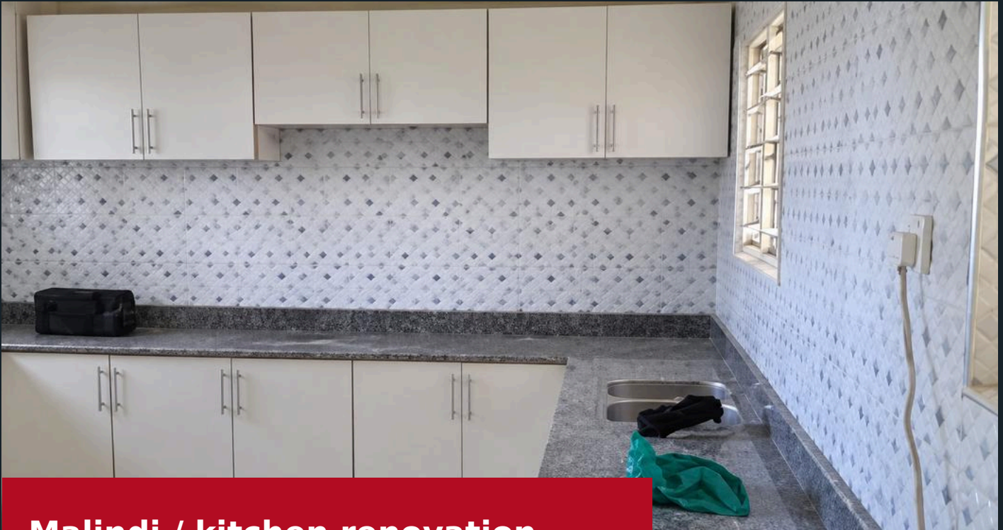
Malindi / kitchen renovation
