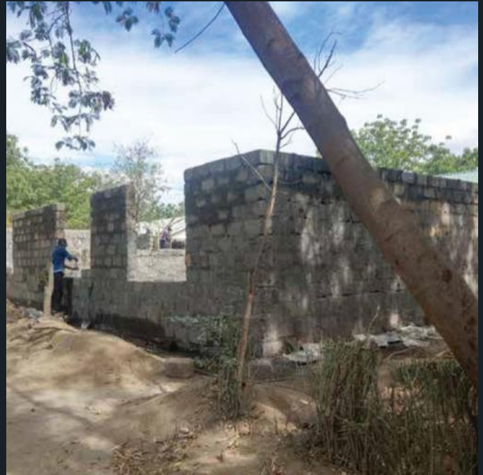
Classroom masonry / Kajiado County
