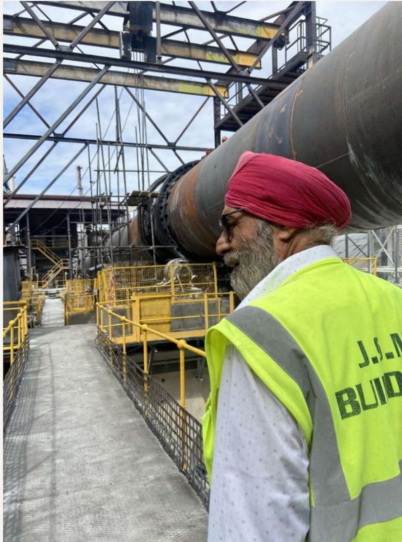
Calcliner shutdown works
