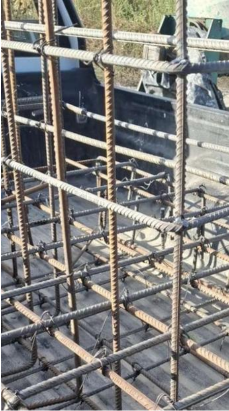
Structural reinforcement / preparation
