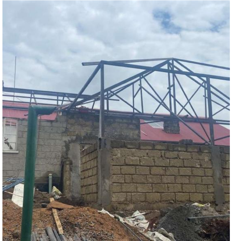
Central Hospital / roof and masonry works
