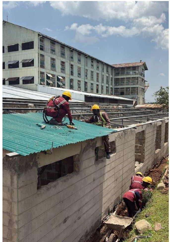
Roof works / steel and sheet interfaces
