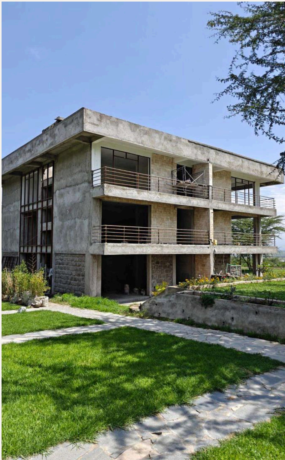
Elementaita house / renovation works
