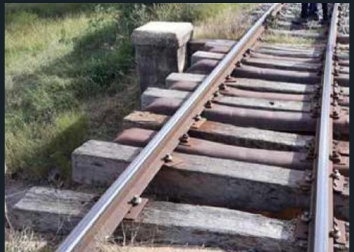
Railway works / track and support structure
