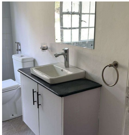
Basin, cabinet and tile junctions
