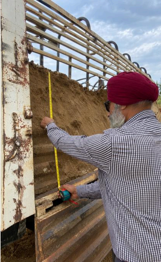
Material delivery verification
