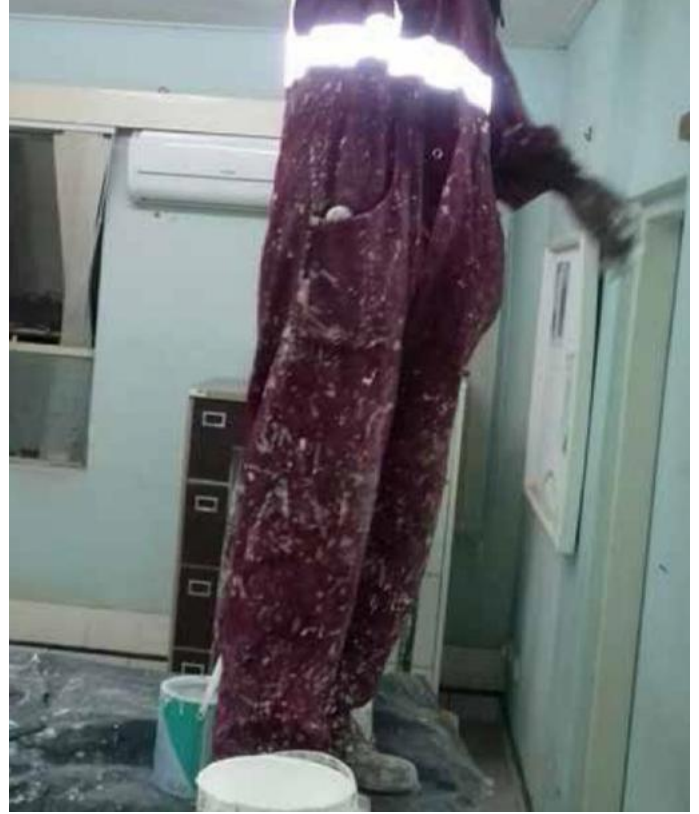
Procurement offices / internal painting
