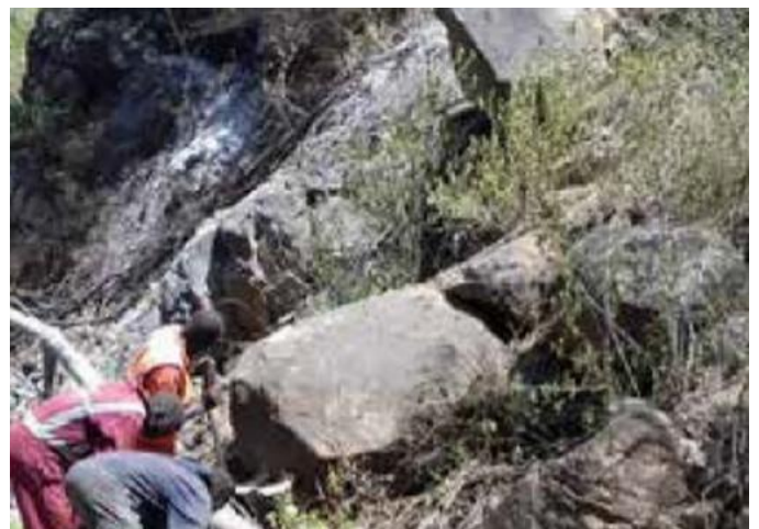
Makueni / water pipeline works
