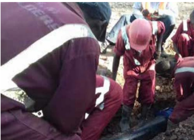
Nyakio / water pipeline works
