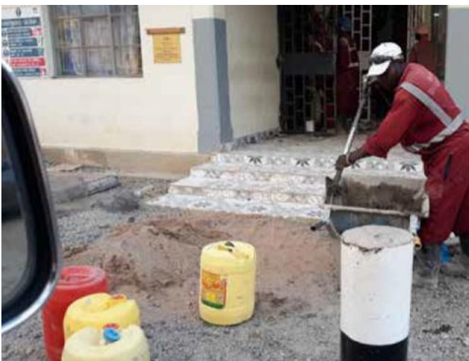
Magadi bank / entrance refurbishment
