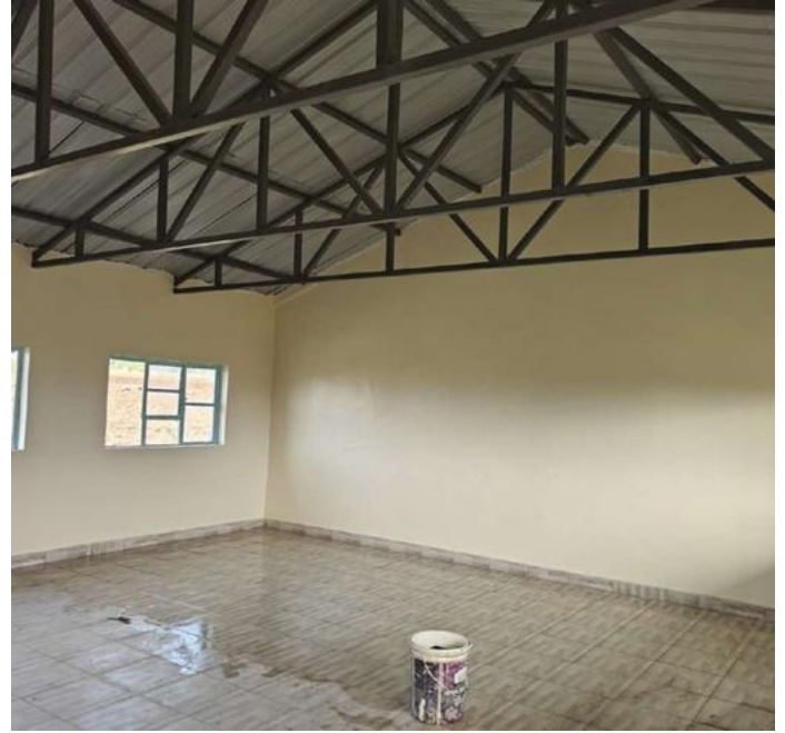
School refurbishment / interior finishes
