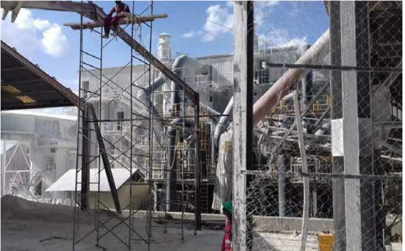
Storage warehouse construction / Tata Chemicals
