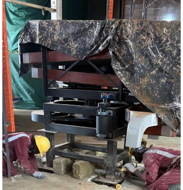
Machine base / anchoring, casting and grouting
