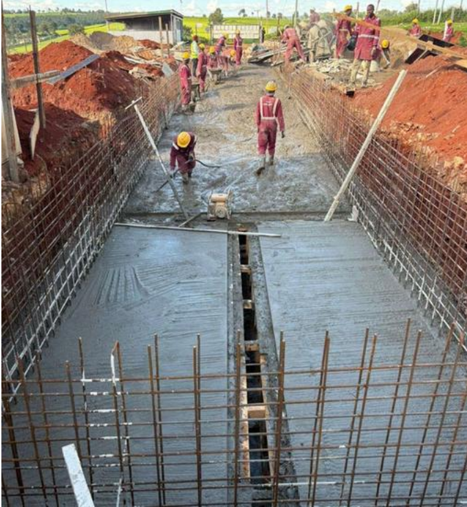
Dispatch ramp / reinforcement and concrete
