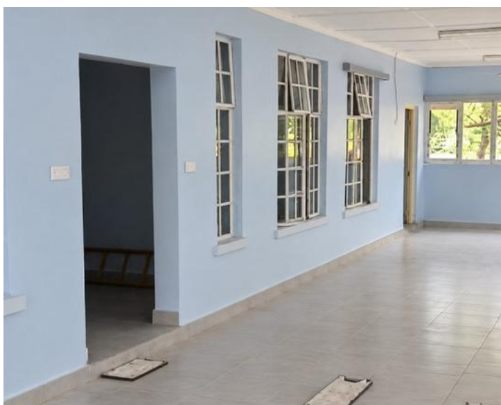
Magadi Soda School / circulation and room finishes
