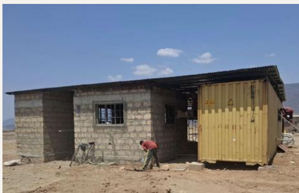
Research lodge / building works
