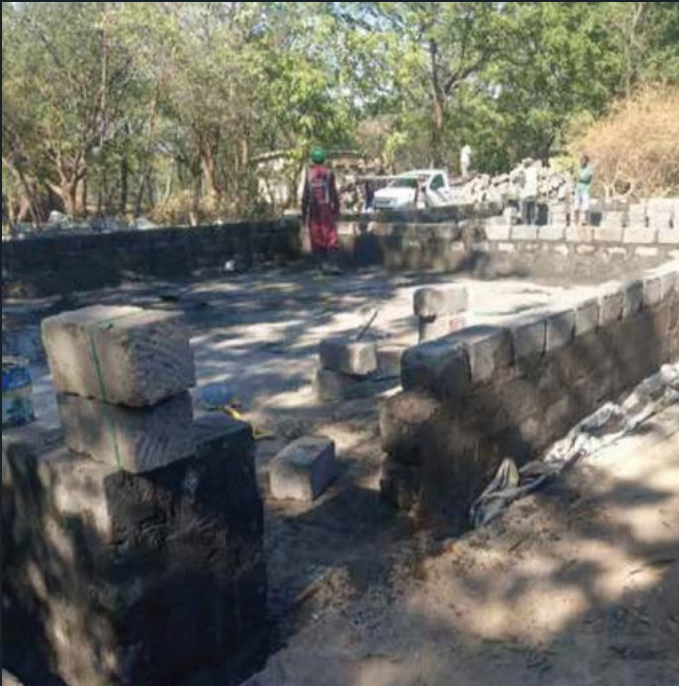
Two-classroom construction / Kajiado County
