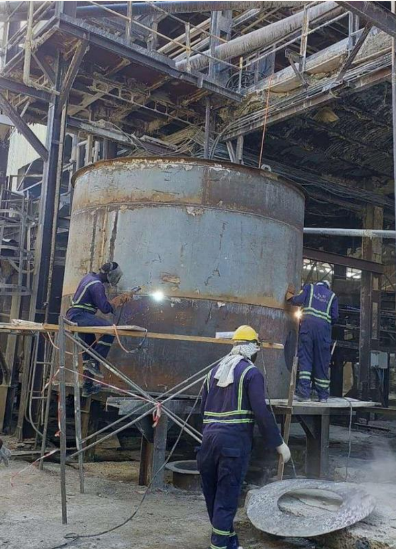
Steel tank fabrication
