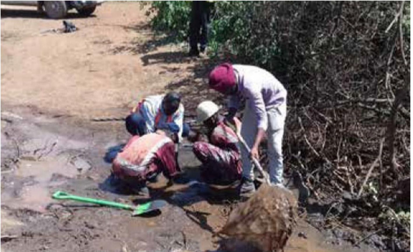
Sampu / pipeline installation
